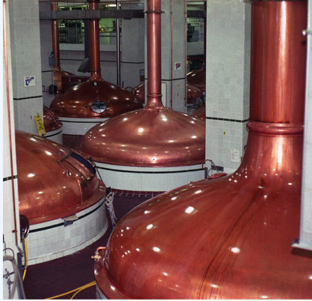
Figure 7.4c: An oxide of carbon is removed from these fermentation tanks through the large copper pipes at the top. (credit: work by Dual Freq, CC BY-SA 3.0)
