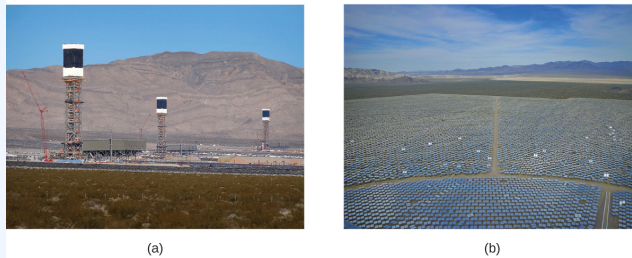
Figure 4.2i: (a) The Ivanpah solar thermal plant uses 170,000 mirrors to concentrate sunlight on water-filled towers. (b) It covers 4000 acres of public land near the Mojave Desert and the California-Nevada border. (credit a: modification of work by Craig Dietrich, CC BY 2.0; credit b: modification of work by USFWS Pacific Southwest Region, CC BY 2.0)
