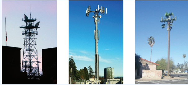
Figure 10.1d: Wireless communication: Radio and cell towers are typically used to transmit long-wavelength electromagnetic radiation. Increasingly, cell towers are designed to blend in with the landscape, as with the Tucson, Arizona, cell tower (right) disguised as a palm tree. (credit left: modification of work by Sir Mildred Pierce, CC BY 2.0; credit middle: modification of work by M.O. Stevens, CC BY 3.0; credit right: work by Gary Minnaert, PD)
