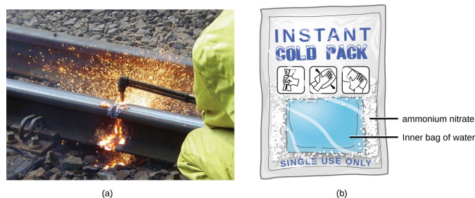
Figure 4.2f (a) An oxyacetylene torch produces heat by the combustion of acetylene in oxygen. The energy released by this exothermic reaction heats and then melts the metal being cut. The sparks are tiny bits of molten metal flying away. (b) A cold pack uses an endothermic process to create the sensation of cold. (credit a: modification of work by Skatebiker, PD; credit b: Chemistry (OpenStax) , CC BY 4.0).
