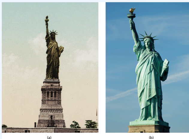
Figure 18.6a (a) The Statue of Liberty is covered with copper skin, and was originally brown, as shown in this painting. (b) Exposure to the elements has resulted in the formation of the blue-green patina seen today. (credit a: work published by Detroit Photographic Company, PD; credit b: work by Dominique James, CC BY 2.0)
